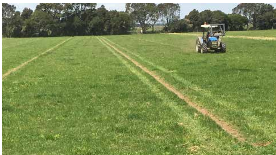
Installing in-field spinner drains.
