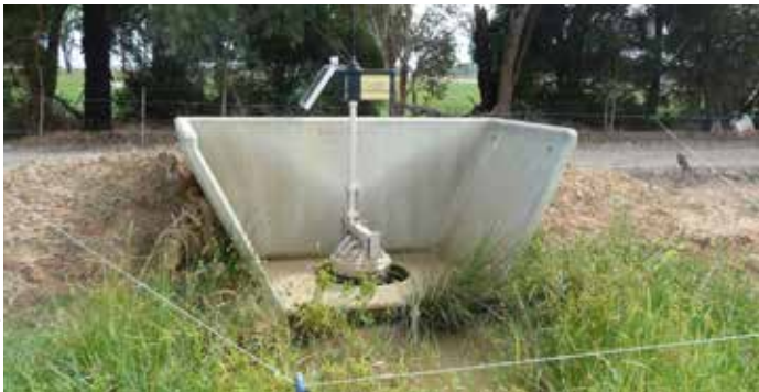
Automated outlet riser from a pipe source.
