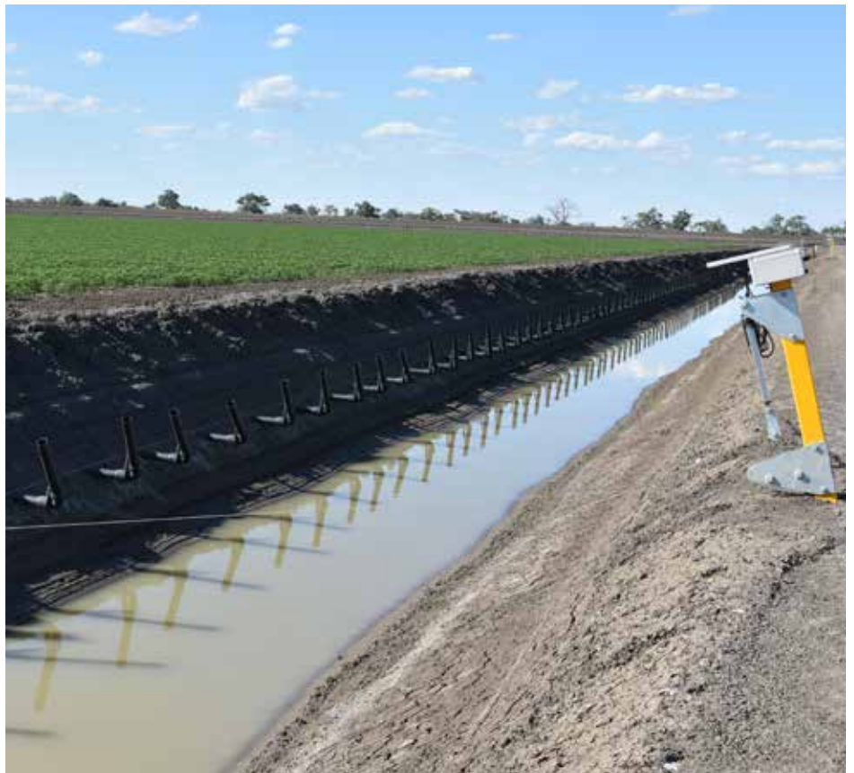
Smart siphons – small Pipe Through the Bank irrigation system.
