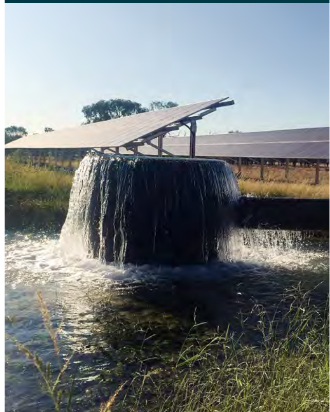
FIGURE 9.3 An industry first installation of a 55 kw submersible pump driven by combined 100 KW solar and 110 kVA diesel generator at the Gill family's 'Waterloo' Narromine, NSW. © Jon Welsh
